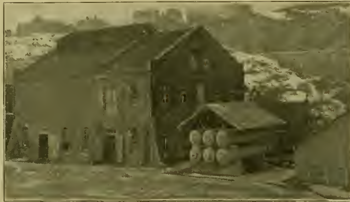
Fig. 1.—Exterior View of Plant.
